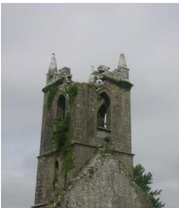
Before: works on the Bell Tower in Former Church in Monivea
