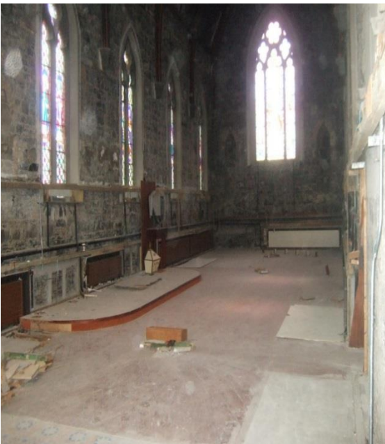
The former convent chapel with the mid-20 th century insertions stripped out
