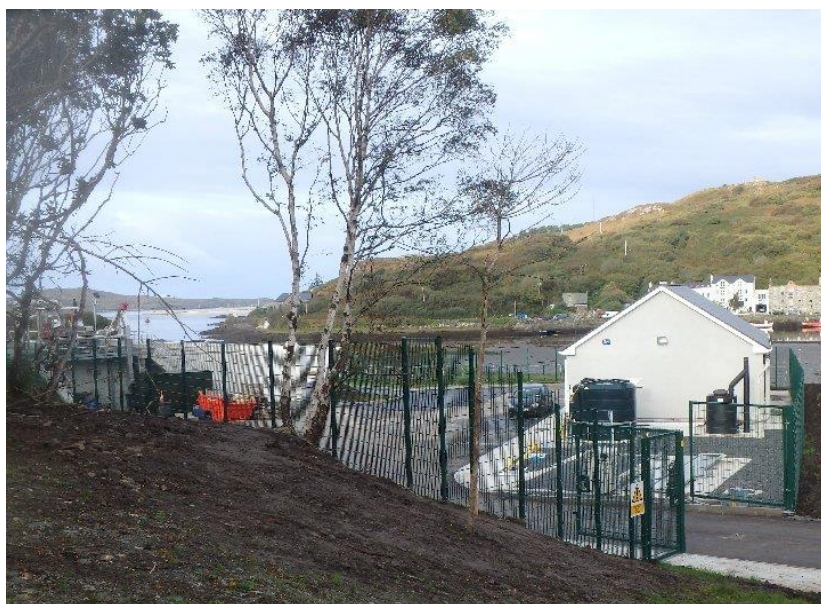
Clifden Waste Water Treatment Plant, Ardbear.
