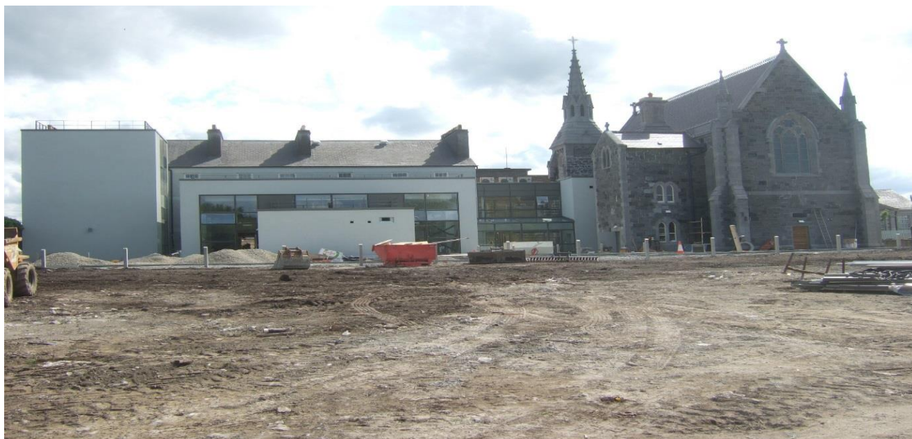
Works ongoing at Ballinasloe Library
