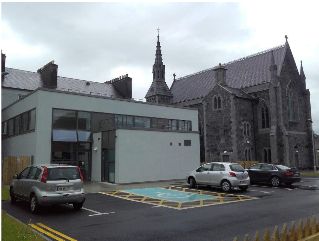
Completed works at Ballinasloe Library
