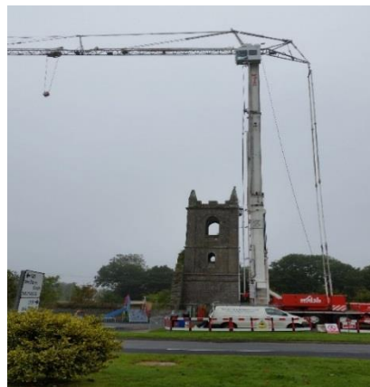
During: the works on the Bell Tower on the Former Church in Monivea
