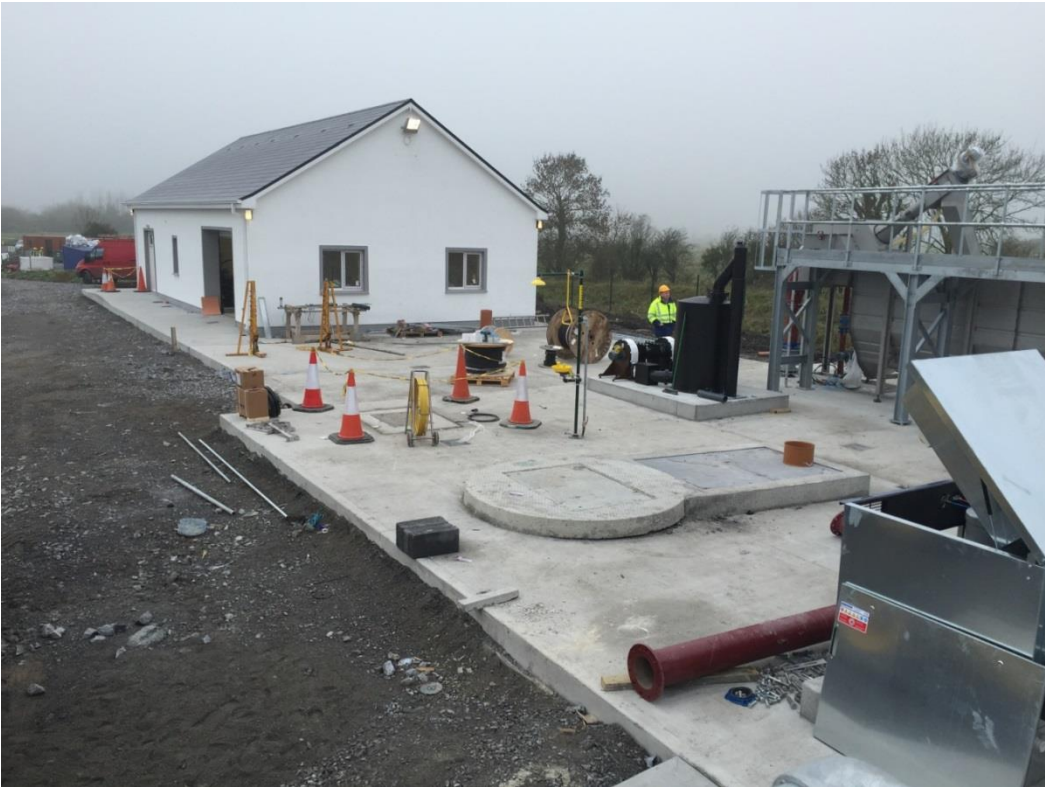
Control Building & Inlet Works at Claregalway WWTP
