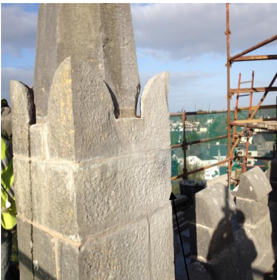
SW pinnacle - stone graft repair almost invisible
