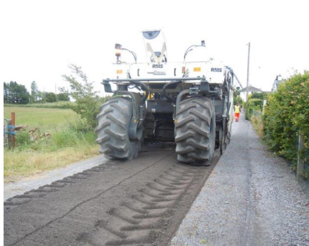
Road re-cycling works at Polldarragh, Tuam
