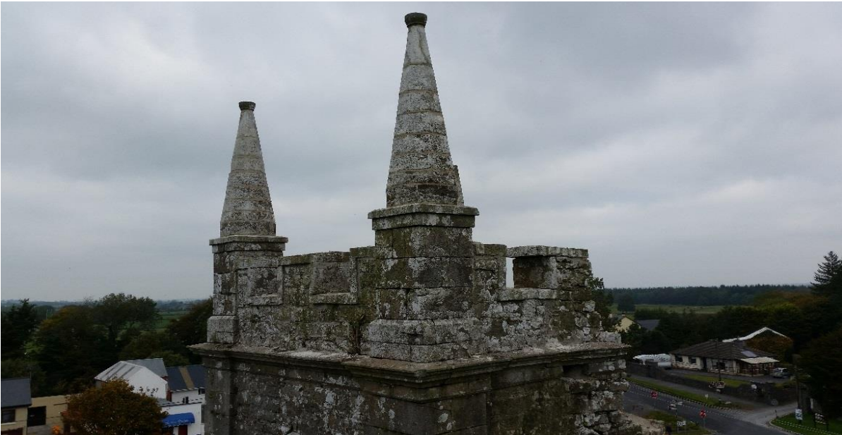
Monivea Bell Tower - Stonework stabilised and secured for the future
