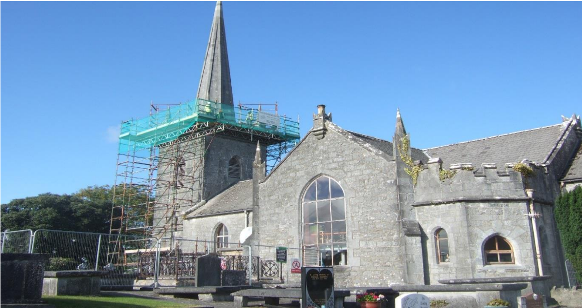
Repairs to parapets and pinnacles
