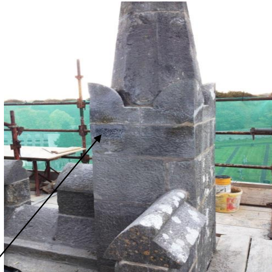
SW pinnacle - stone graft repair almost invisible
