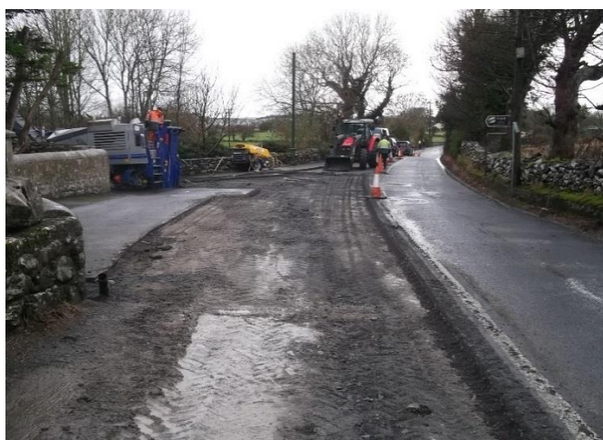
Road resurfacing on the Maree Road, Oranmore
