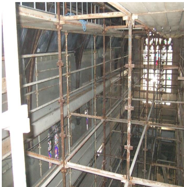
During: Scaffolding erected to allow access to facilitate repair of the painted plaster panels of the interior of the roof
